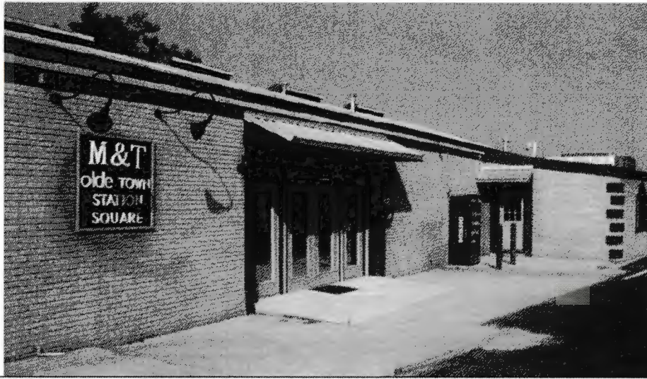
TYPICAL VIEW OF THE SUBJECT PROPERTY
